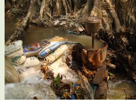
Rev. Lazarus explains that channels providing a necessary flow of water for external turbine units should measure approximately 1 ft. deep by 1 ft. wide (0.3 m x 0.3 m) for 1 kw micro-hydro units. Larger 2 kw units require 2 ft. x 2 ft. (0.6 m x 0.6 m) channels, whereas slightly larger channels are needed for 3 kw generators.
