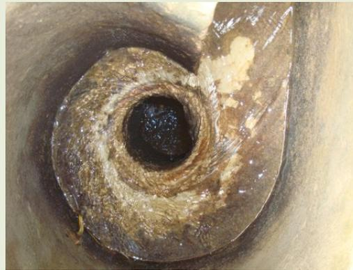
The most important component of such channels is a feature that forces water to ultimately spin in a clockwise vortex which in turn causes the external turbine of a micro-hydro unit to rotate. To enable the vortex effect, the end of the channel should be rounded and include a minimal 5-6 inch (12.7 cm - 15.2 cm) intake opening through which water can spin into the top of a cement or PVC penstock (a vertical drainage shaft).
