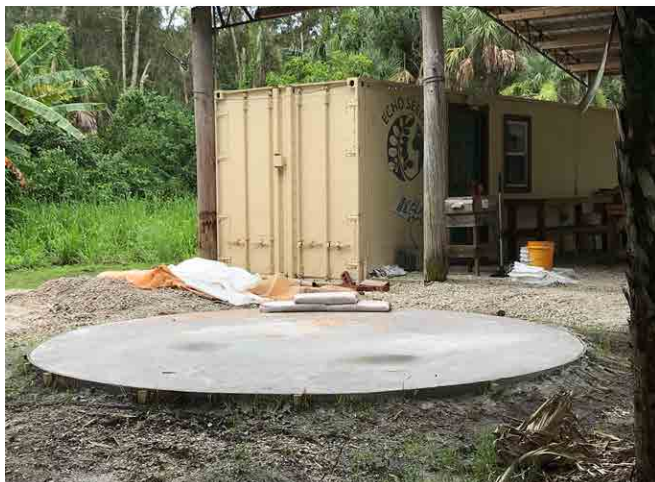
Figure 2. ECHO Florida's concrete slab foundation for an earthbag seedbank (left), and an illustrated cross-section (right).
