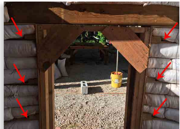
Figure 11. Arrows indicate velcro plate placement after every third course. Source: Tim Motis.
