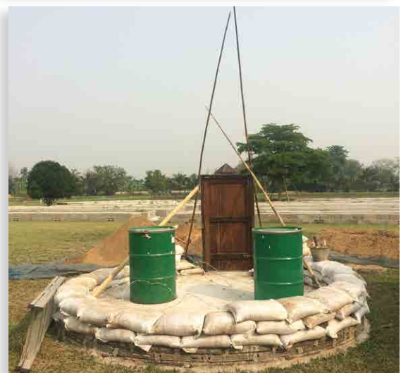
Figure 3. The door forms in place at ECHO's Florida location (left) and Thailand office (right). Source: Cody Kiefer (left) and Patrick Trail (right).
