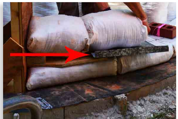
Figure 9. Close up of slider use in bag placement. Source: Tim Motis.
