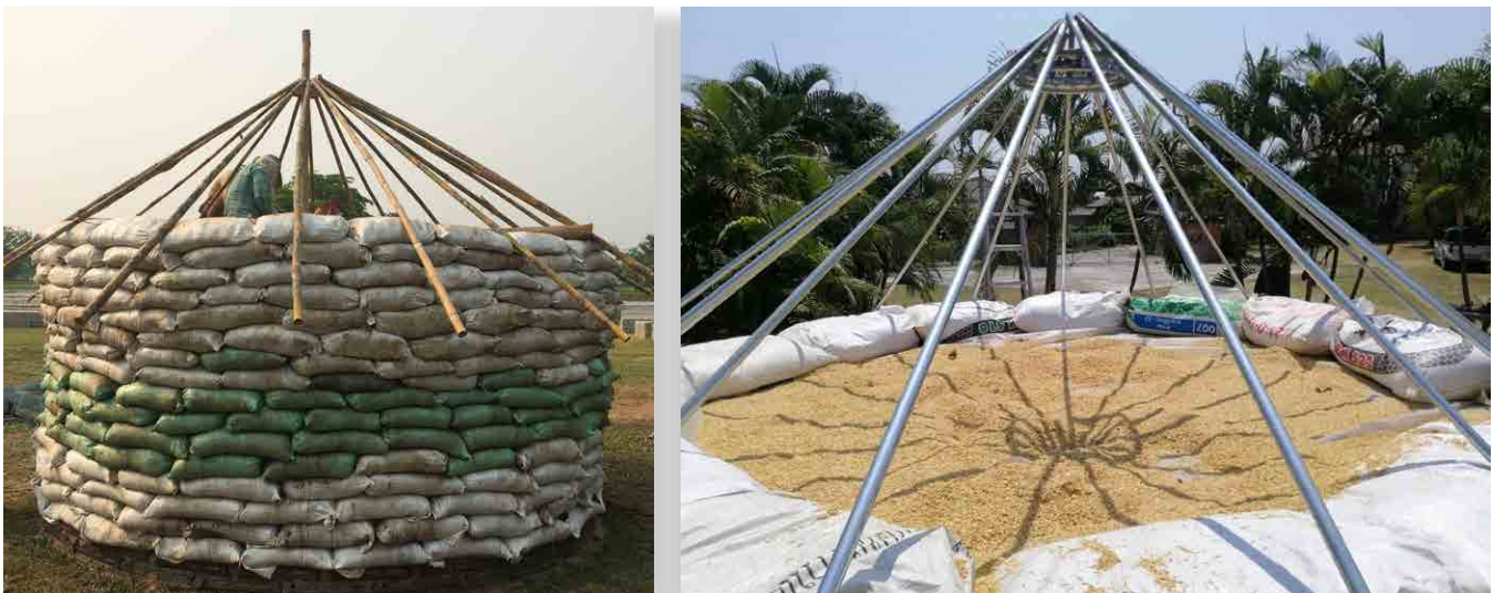
Figure 13. ECHO's Thailand office initially installed a bamboo-based roof structure (left) and was later replaced with a metal structure (right). Source: Patrick Trail.
