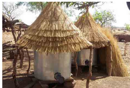
Figure 12. Finished metal silos roofed to protect them from the elements. Source: Edward Martin
