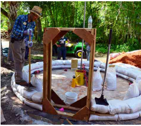
Figure 7. Tamping bags to form walls of an earthbag house. Source: Cody Kiefer
