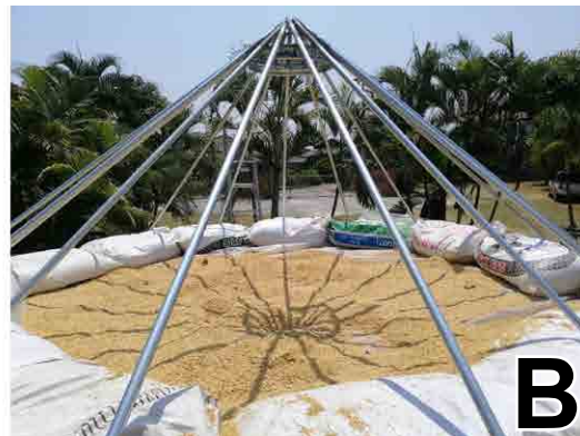
Figure 10. Bamboo (A) and metal (B) as options for rafters. Note rice hulls placed on top of plywood ceiling for insulation. Source: ECHO Asia staff
