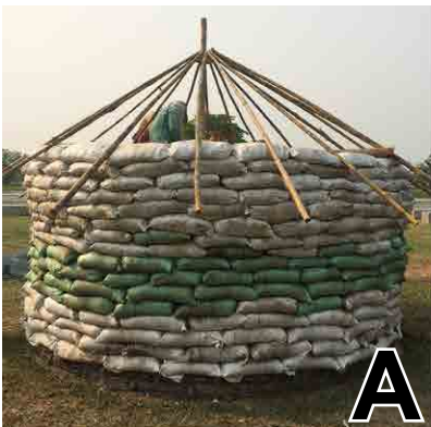
Figure 10. Bamboo (A) and metal (B) as options for rafters. Note rice hulls placed on top of plywood ceiling for insulation. Source: ECHO Asia staff
