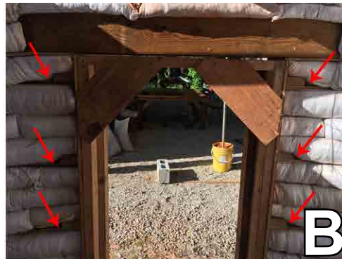
Figure 9. Wooden anchor (A), between every third layer of bags (B), to which the doorframe was attached. Source: Cody Kiefer (A) and Tim Motis (B)
