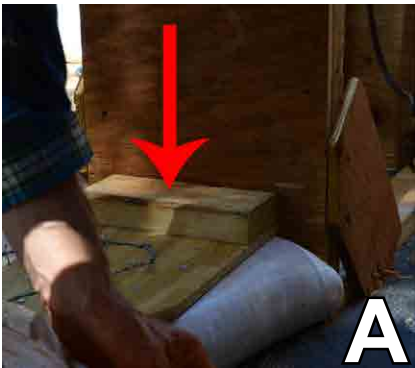
Figure 9. Wooden anchor (A), between every third layer of bags (B), to which the doorframe was attached. Source: Cody Kiefer (A) and Tim Motis (B)
