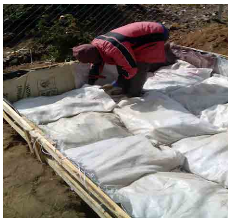
Figure 1. Incorporating fill material into water reservoir of a 100-fold garden. Source: Lance Edwards
