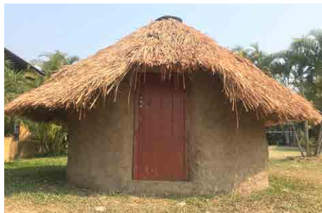
Figure 2. Earthbag house at ECHO in Thailand. Source: ECHO Asia Staff
