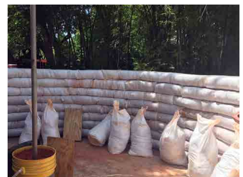
Figure 6. Pole for measuring distance of each bag from the center of a circular earthbag house. Source: Cody Kiefer
