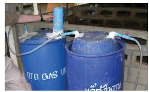
Seal the area between the pipe and the lid with waterproof epoxy sealant or any other tight sealing method.
