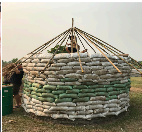
Figure 5: Earth-bag seed storage room under construction at the ECHO Asia Small Farm Resource Center. Bags are partially filled with rice hulls.
