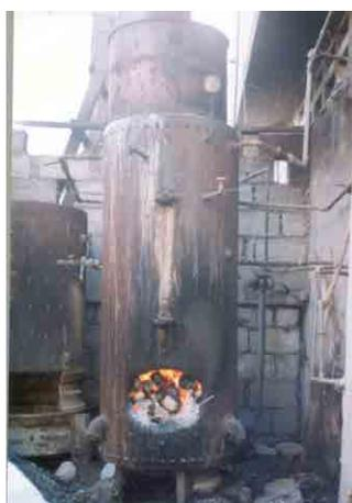
**Figure 11:** Burning briquettes to heat water for a dry cleaning business.
