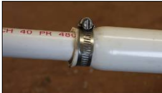
1.25" pipe compressed onto 3/4" pipe with hose clamp
