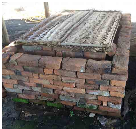
Figure 8. An evaporative cooling chamber at AVRDC in Tanzania, made with bricks. Source: Stacy Swartz
