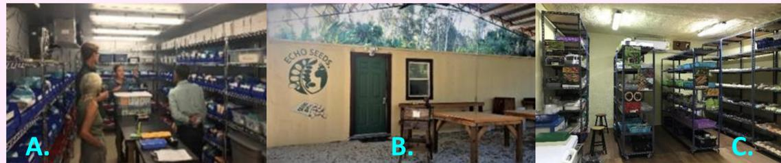
Figure 1. (A) ECHO Global Farm Seed Bank Cold Room, climate-controlled for temperature and humidity. (B) ECHO Global Farm Container Cold Room, retrofitted refrigerated shipping container. (C) ECHO Asia Impact Center, foam insulated split-unit A/C cold room.
