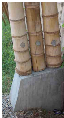
Figure 18. Bamboo posts secured to a concrete footing internally with steel, and hollow internodes infilled with concrete (left). A fishmouth being joined using a steel eye-bolt (right). Source: Craig Bielema
