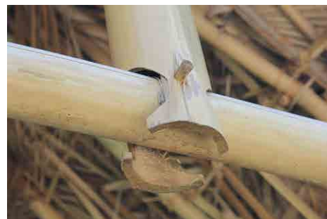
Figure 11. 'Through mortise and tenon': A smaller diameter bamboo passing through a mortise cut through both walls in a larger diameter bamboo. Source: Craig Bielema
