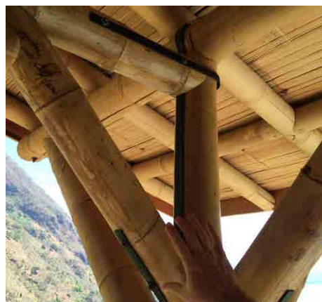
Figure 19. A bamboo hotel in Guatemala, most of the joints are made using steel straps and bolts. Source: Craig Bielema
