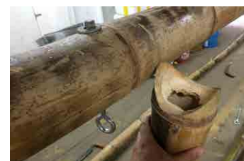
Figure 18. Bamboo posts secured to a concrete footing internally with steel, and hollow internodes infilled with concrete (left). A fishmouth being joined using a steel eye-bolt (right). Source: Craig Bielema
