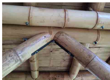
Figure 19. A bamboo hotel in Guatemala, most of the joints are made using steel straps and bolts. Source: Craig Bielema
