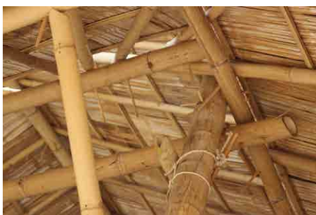
Figure 17. Bamboo peg used to join bamboo poles together. Source: Craig Bielema
