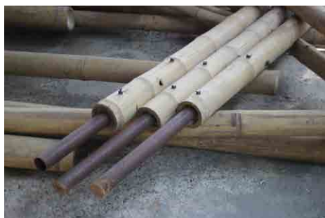
Figure 12. Bamboo fitted with steel 'loose tenons' which are secured in place with bolt. Source: Craig Bielema
