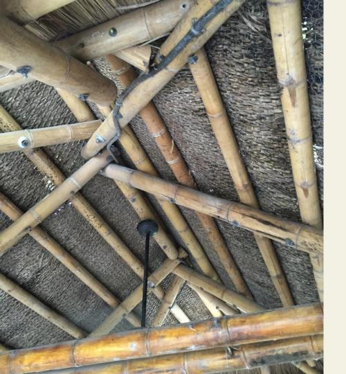
Treated bamboo is an excellent material for housing construction.
