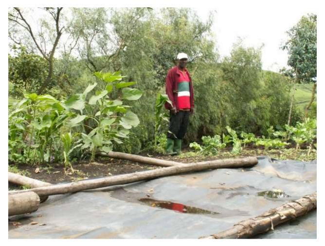
A hafir is a trench lined and covered with plastic sheeting costing around 100 USD. It is a home water cistern filled by rain surface water from the ground or from the house roof or a well-designed trench. It is very practical in highland.
